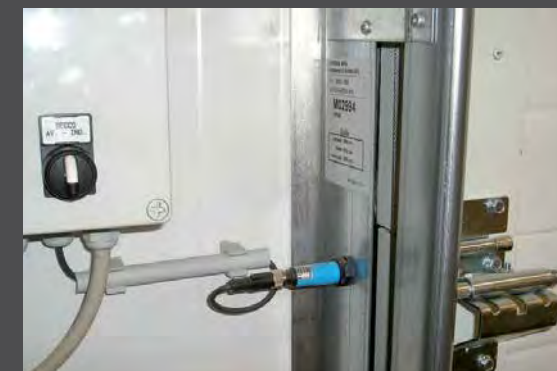
SENSORE PER INTERCONNESSIONE RAMPA-PORTONE DOCKLEVELLER-DOOR CONNECTING SENSOR
